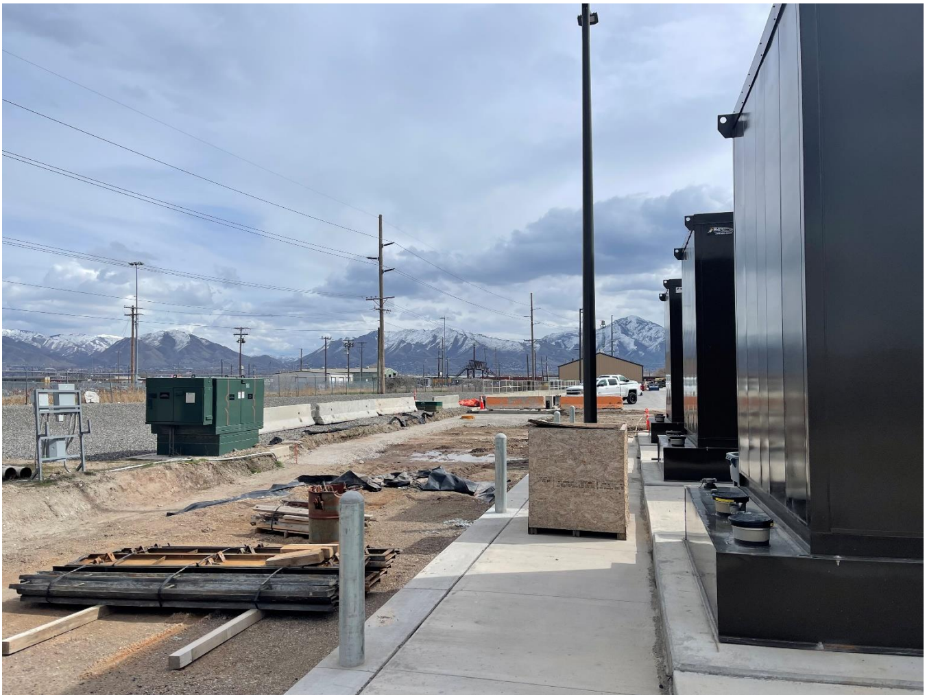
Grading for Asphalt, North of Generators. Looking East.
