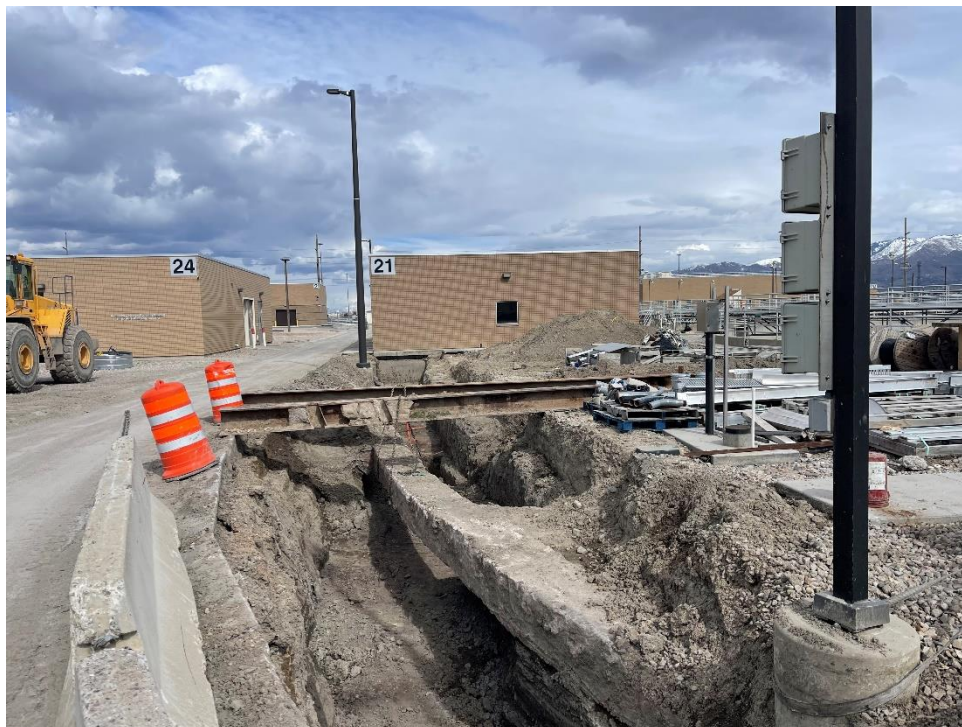
RAS Piping Excavation, East RAS, looking North.
