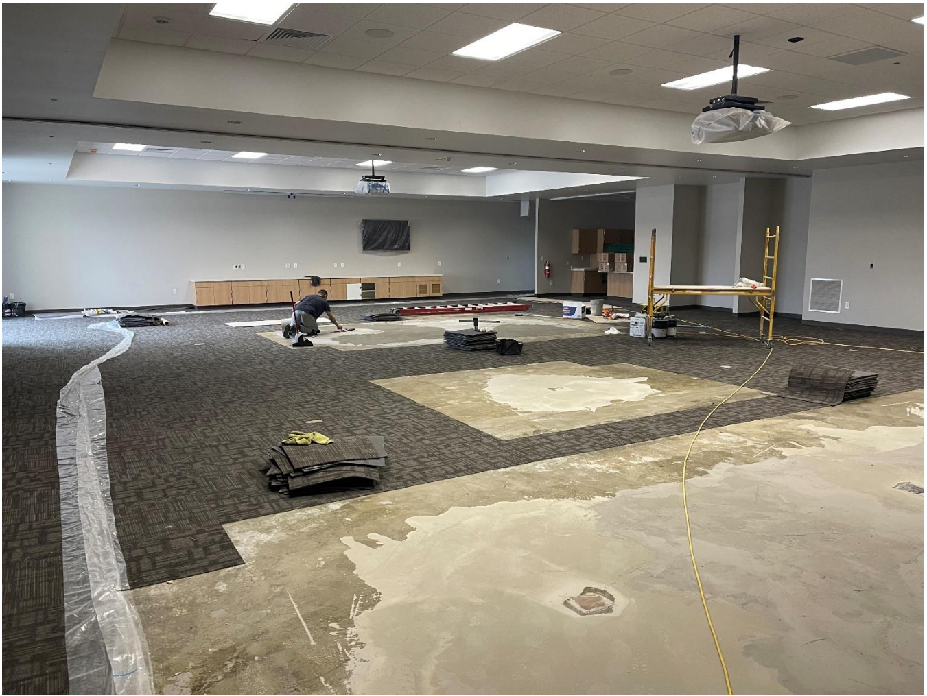
Training/Conference Room, Looking Southwest
